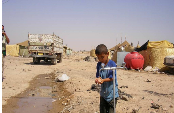
Installation of Water Network in Manathera Camp: © IOM/2007
